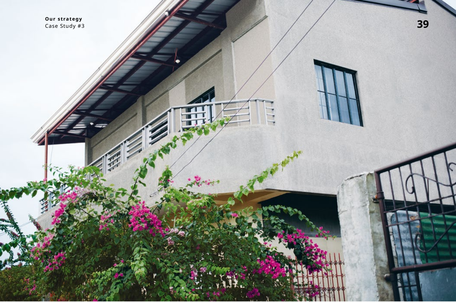
Nida Santa Romana's house is in the finishing stages of construction.
