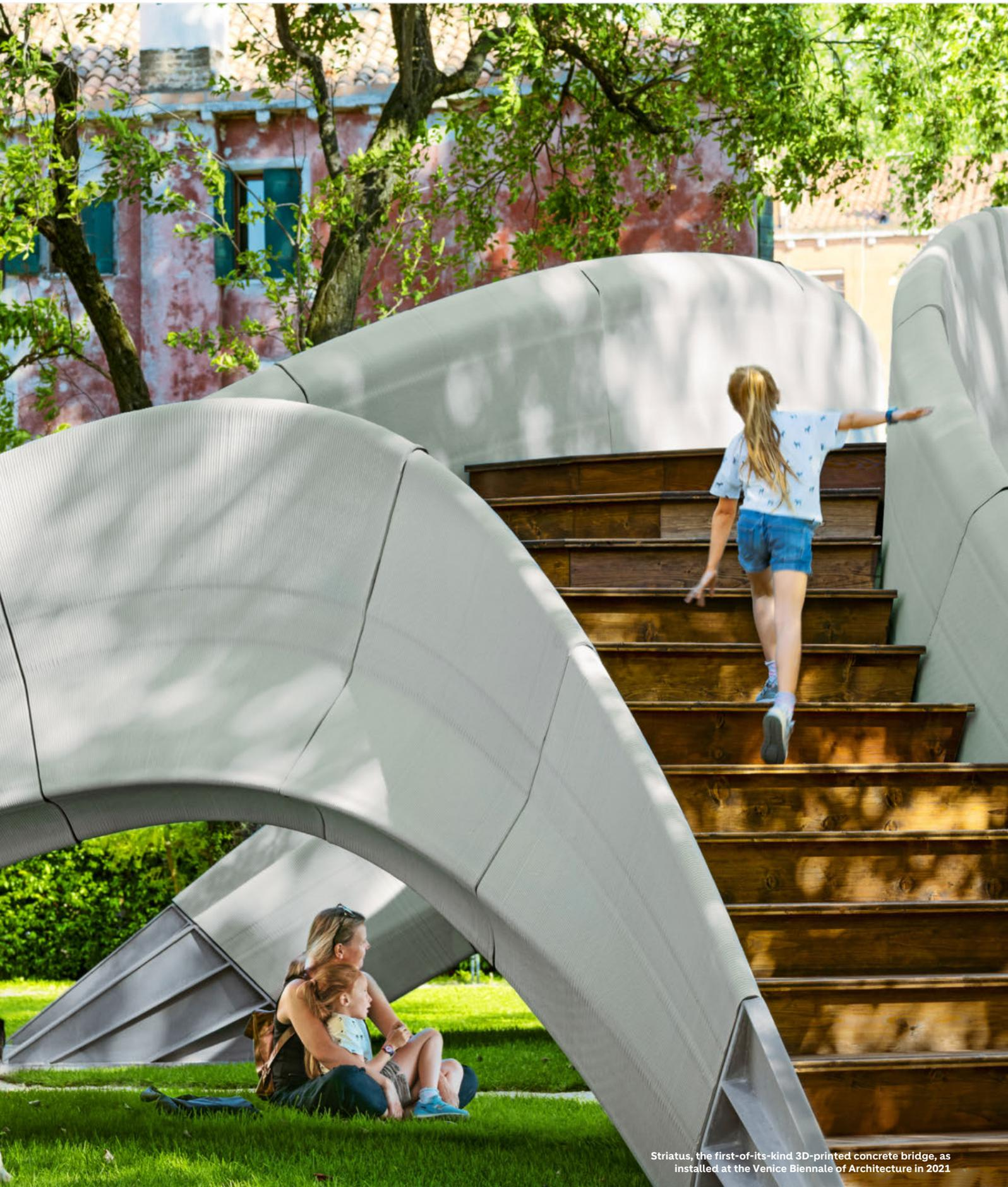
Striatus, the first-of-its-kind 3D-printed concrete bridge, as installed at the Venice Biennale of Architecture in 2021
