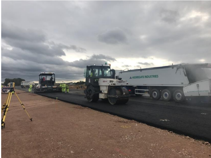
Photo: A14 works
