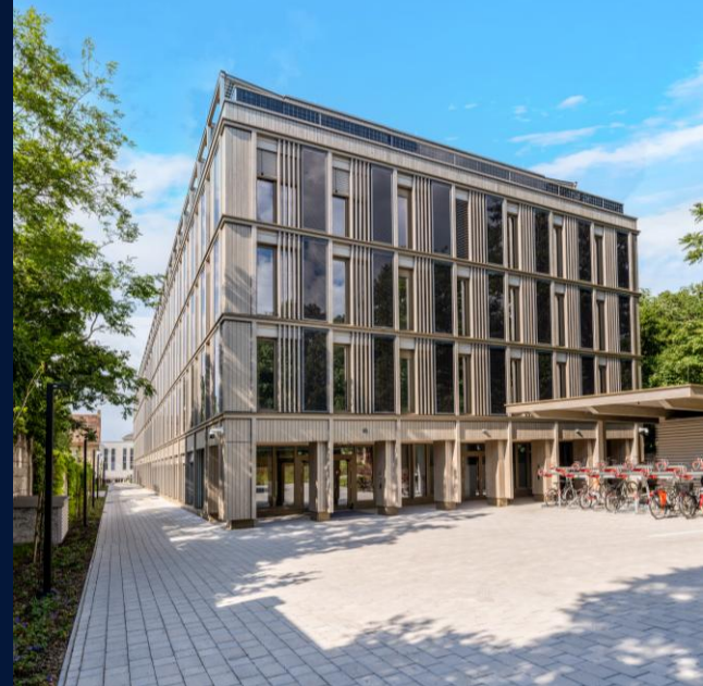
European Patent Office in Vienna, Austria Built with ECOPact with ECOCycle inside, and Isoguard
