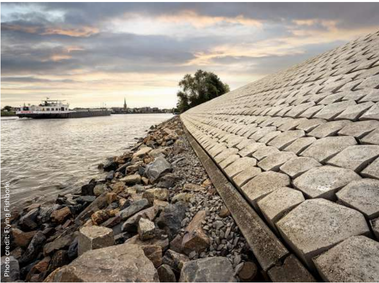
Basalton Quattroblock revetment, Nieuwekerk, The Netherlands
