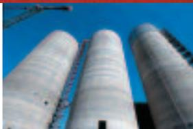
Doumit Saadé has every reason to smile. The three cement silos, each designed for a capacity of 12,000 tonnes, are almost complete. "We are on track as planned. It is a fascinating project!"
