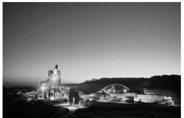
The new Ste. Genevieve plant of Holcim US in Missouri.
