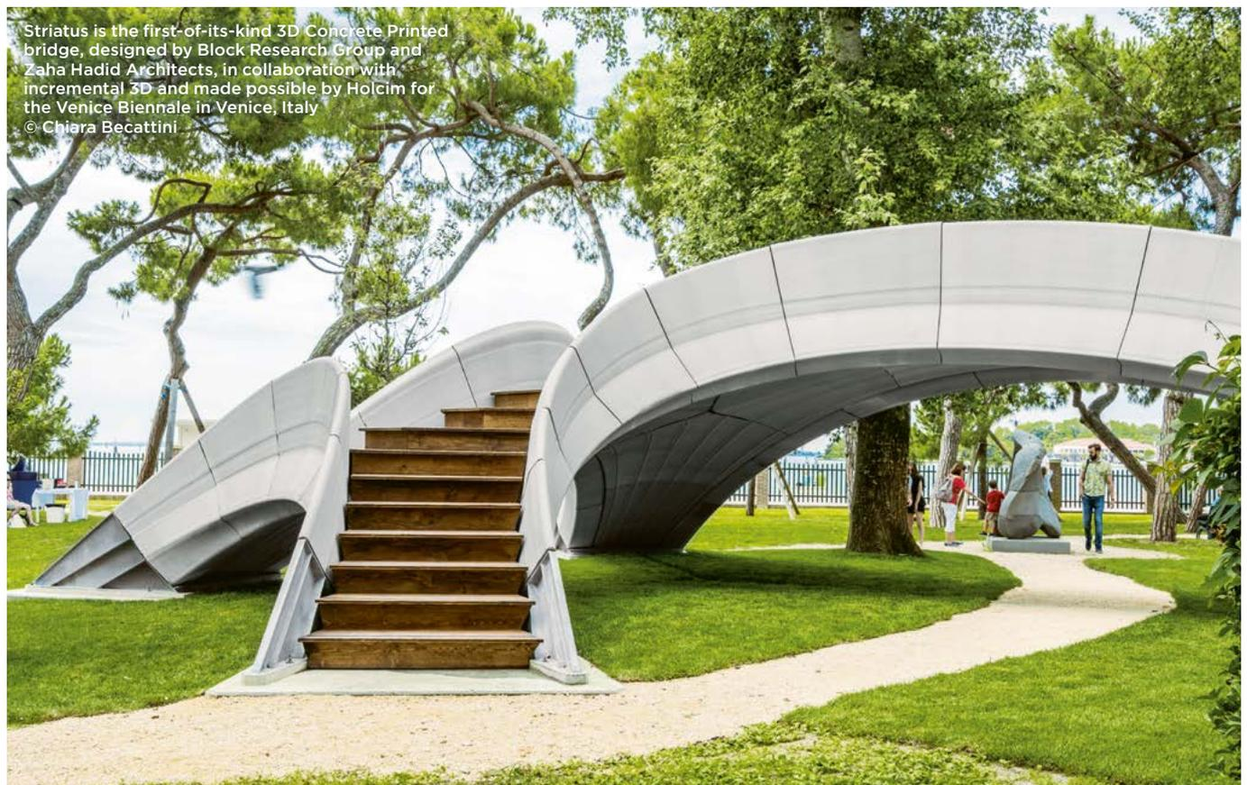
Striatus is the first-of-its-kind 3D Concrete Printed bridge, designed by Block Research Group and Zaha Hadid Architects, in collaboration with incremental 3D and made possible by Holcim for the Venice Biennale in Venice, Italy
